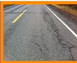
Minor Structural Distress
